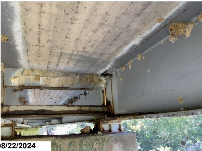
Bent 30 ahead girder 1: heavy flaking rust with section loss near bearing area and haunch. 4LF CS3 Corrosion. Common all girders this location.
