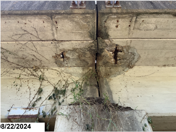
Bent 15 right side overhangs of spans 14 and 15 have exposed rebar. 2' CS3
