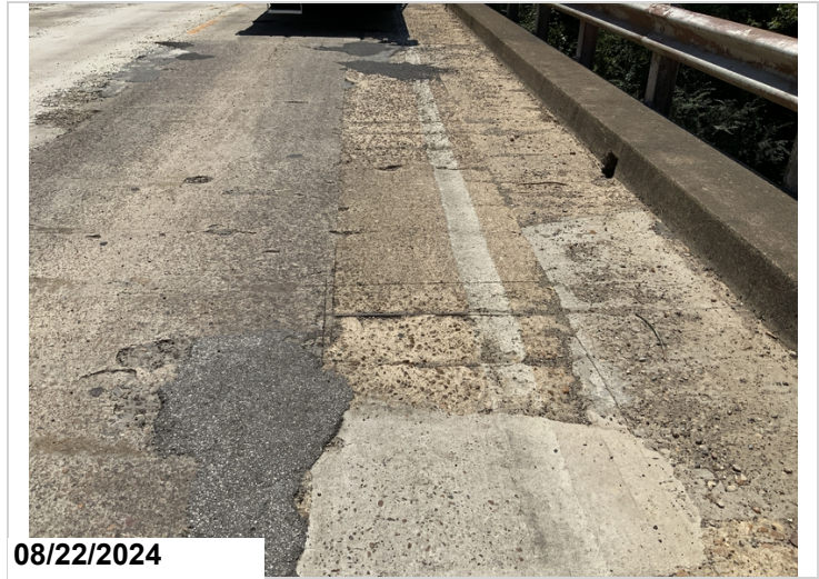
Deck Span 29 near bent 30 right lane: spalls with exposed rebar 20' CS2
