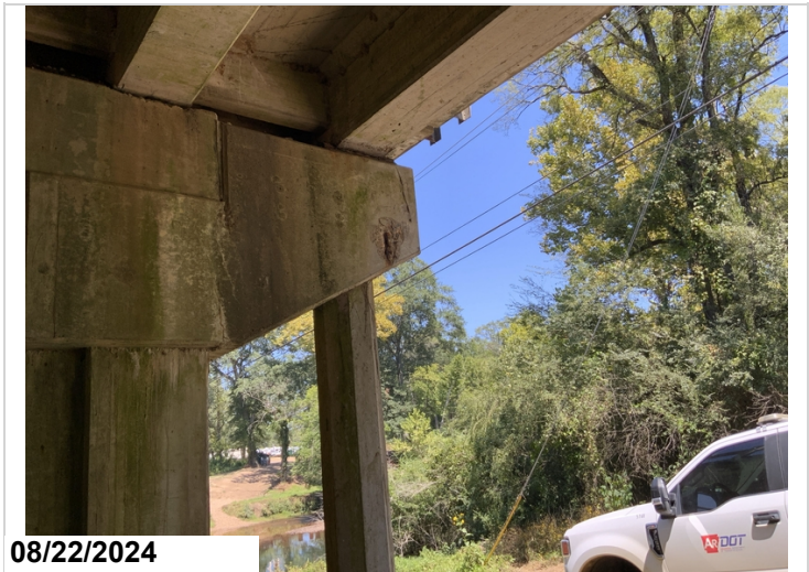
Bent 28 cap back right side exposed rebar CS3 1'
