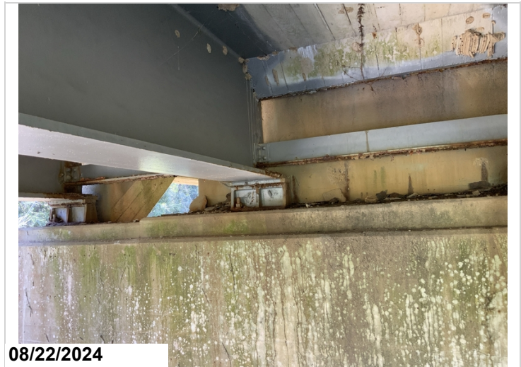
Overview of bent 29 ahead: rust to lower web/ flanges, bearings and diaphragms. 6' CS2
