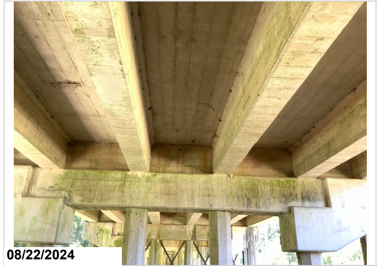
Span 17 bay 2 exposed rebar 3' CS3
