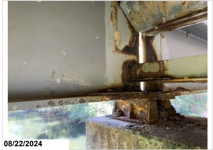
Bent 30 ahead, girder 5: heavy flaking rust with section loss near bearing area and haunch. 4LF CS3 Corrosion.
