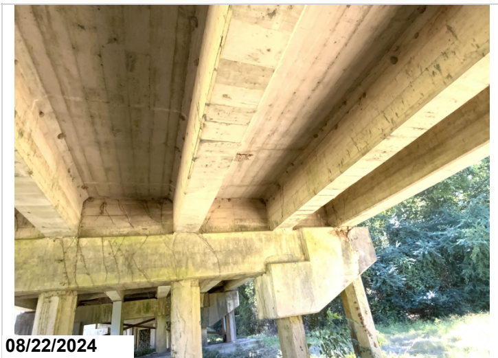
Bent 6 cap ahead left side 1' exposed rebar CS3
