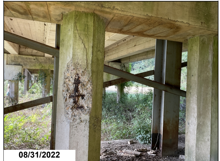
Bt. 15, pile 4, spall with exposed rebar.
