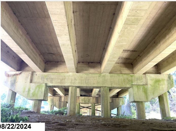
Span 18 bay 2 exposed rebar 6' CS3
