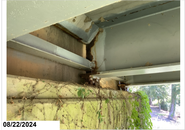
Span 30 bent 31 bearing 4 & 5: flaking and tilted CS2
