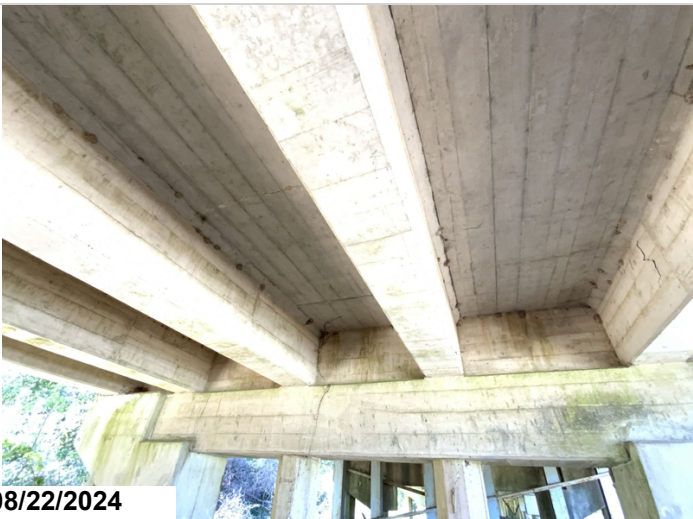
Span 15 all bays have cracks with efflorescence 23' CS2.
