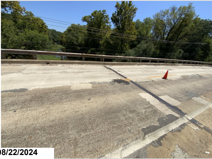
Spans 29 & 30 right lane has patched deck repairs.
