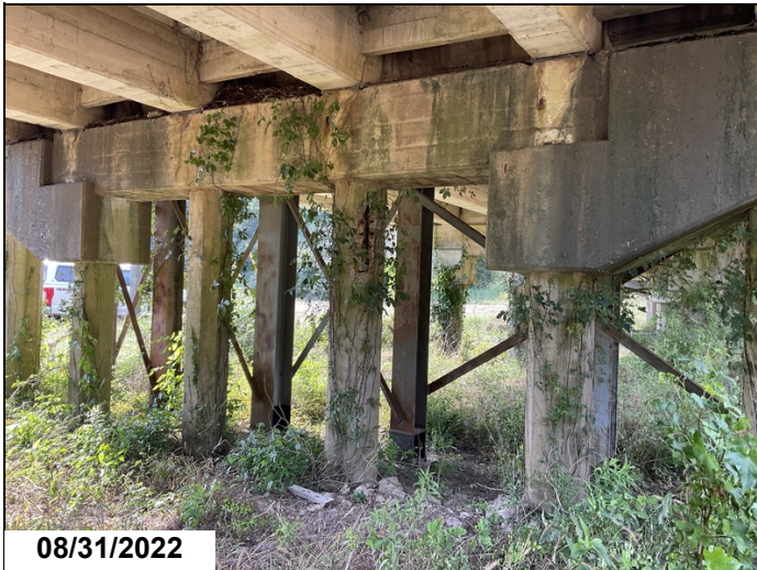
Bent 10, pile 3, spall with exposed rebar.
