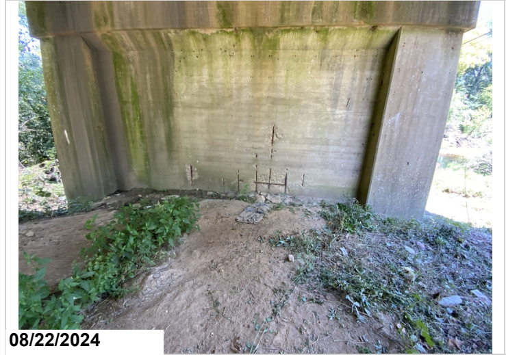
Bent 29 back pier wall 7' exposed rebar CS3
