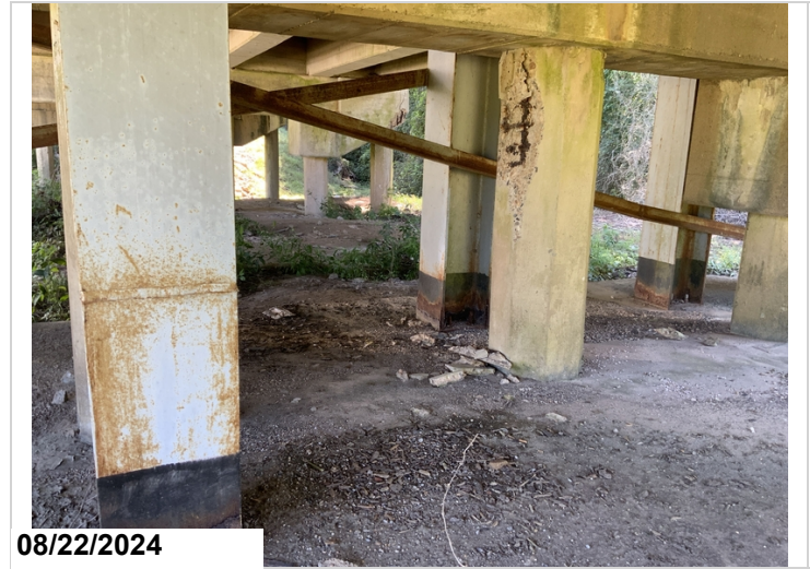
Bent 5 pile 3 exposed rebar CS3
