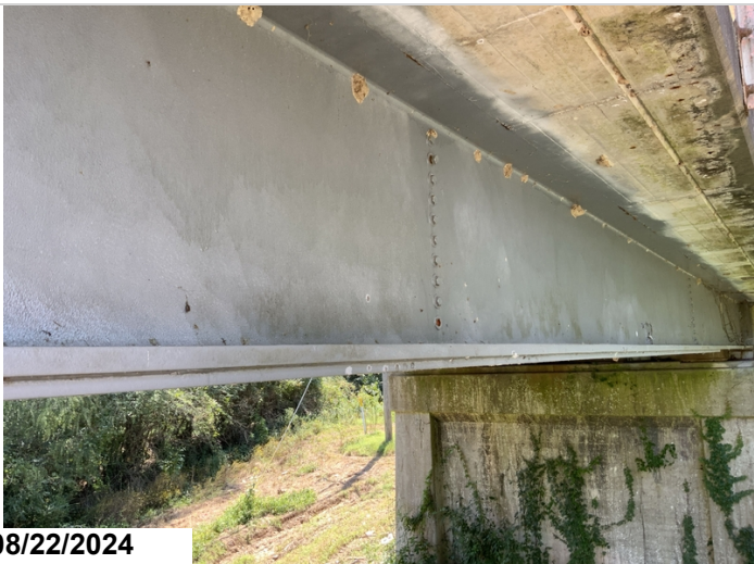
Span 29 girder 1 at second diaphragm ahead of bent 29: missing and broke bolts.
