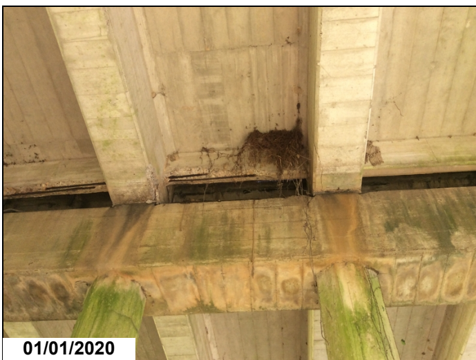
Span 23 at Bt. 24, girders 3 & 4 have spalls.
