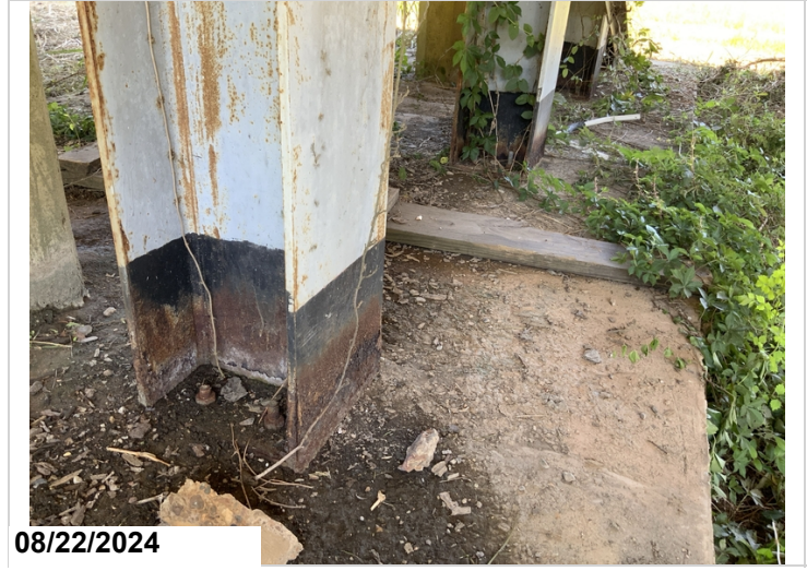
Bent 11 all steel piles have flaking rust 6' CS2
