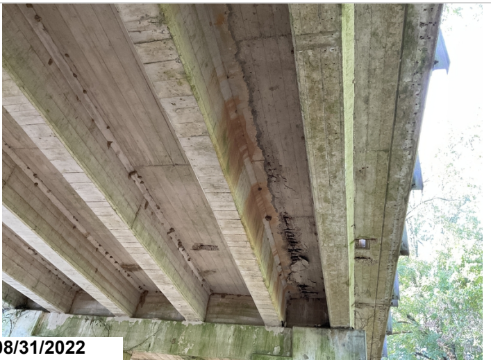
Span 25, bottom side of top flange, spalls with exposed rebar between girders 1 & 2.
