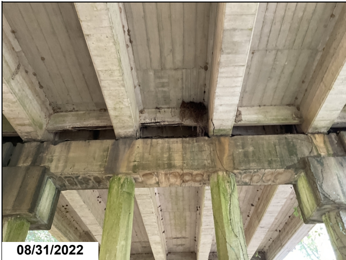
Span 23 at Bt. 24, girders 3 & 4 have spalls.
