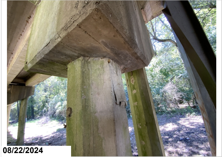
Bent 27 pile 2 has crack and delam CS2
