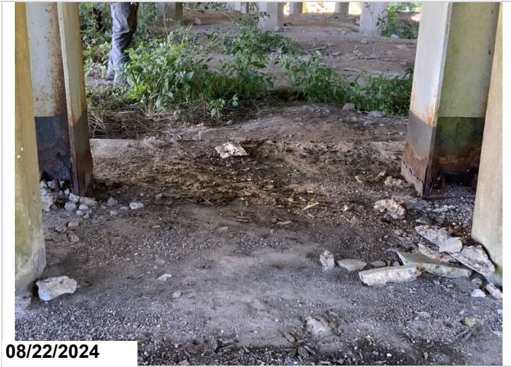
Bent 5 all steel helper piles have flaking rust 6' CS2
