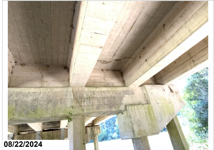
Bent 14 cap ahead left side 1' exposed rebar CS3
