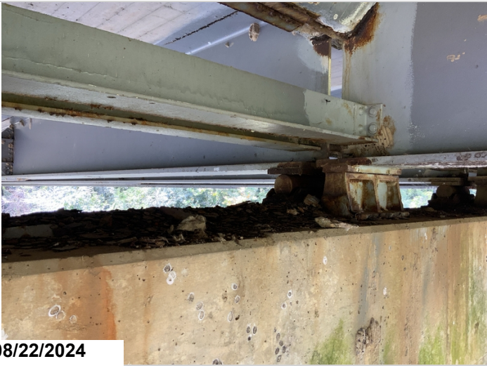
Bent 30 bearings have heavy flaking rust with some debris buildup up CS3
