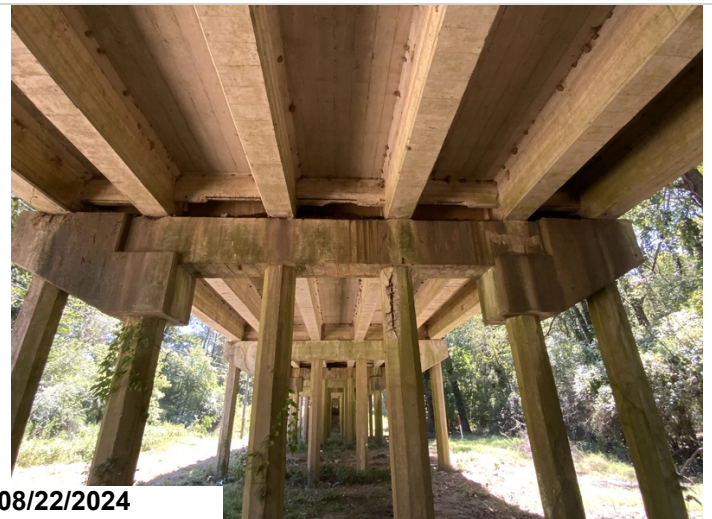
Bent 26 pile 3 exposed rebar CS3
