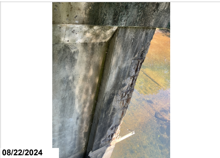
Bent 30 column 2 back: large spall with exposed rebar. CS3
