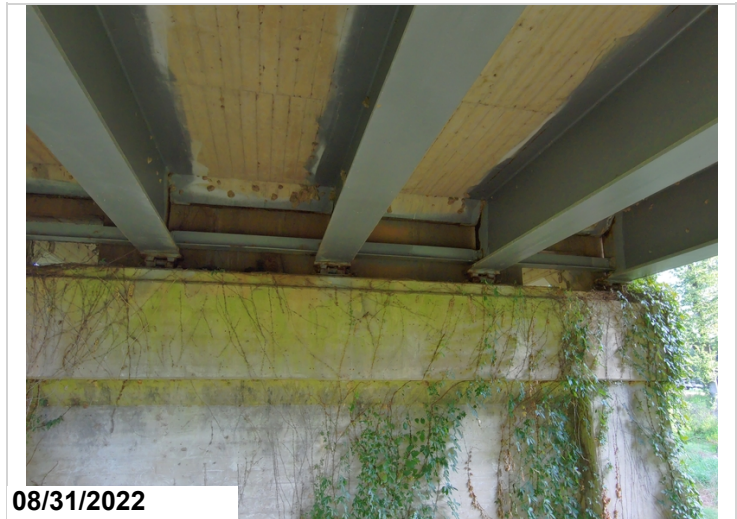
Span 30 at Bt. 29, beam ends have corrosion
