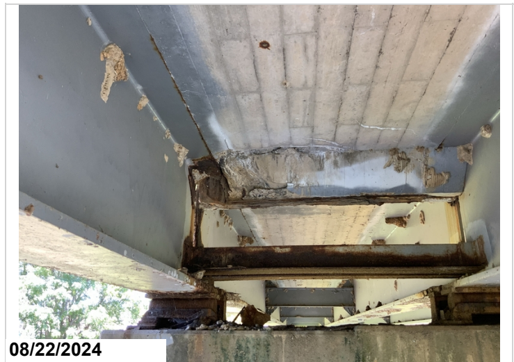
Span 29 bent 30 girder 1 right: heavy flaking rust at haunch CS3
