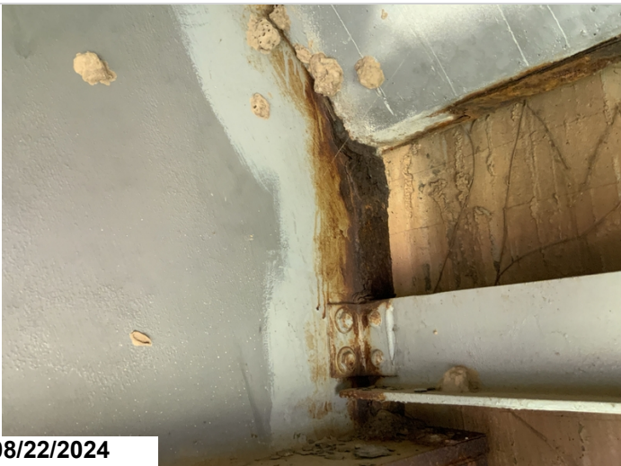
Span 30 bent 31 back girder 2: heavy flaking rust at haunch CS3
