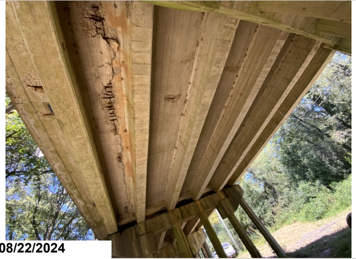
Span 25 bay 1 and left over hang exposed rebar 13' CS3.
