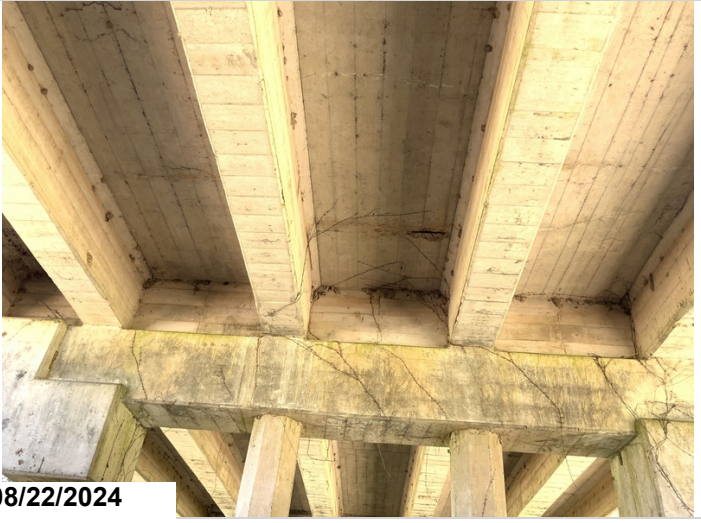
Span 8 all bays have cracks with efflorescence 20' CS2
