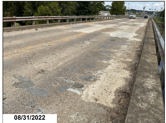
Span 29 & 30, spalls with exposed rebar.
