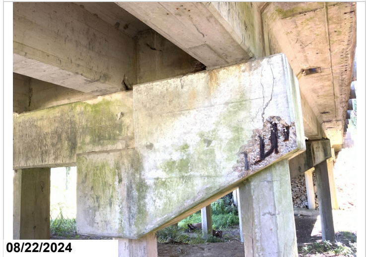
Bent 4 cap ahead left side 1' exposed rebar CS3
