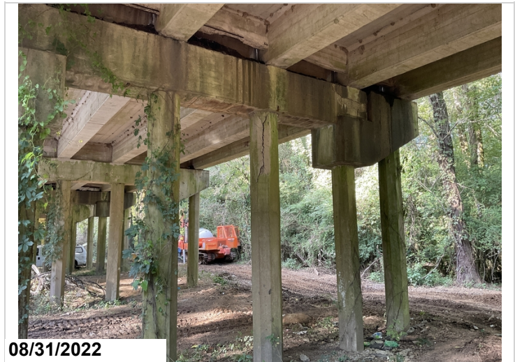
Bt. 26, pile 3 has large crack, cap has spall below girder 2.
