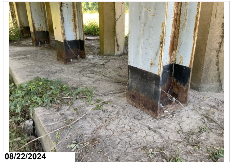
Bent 7 all 6 steel piles have flaking rust 6' CS2
