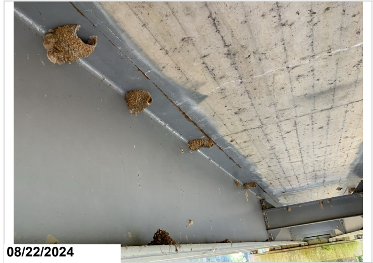
Typical paint system near top flange.
