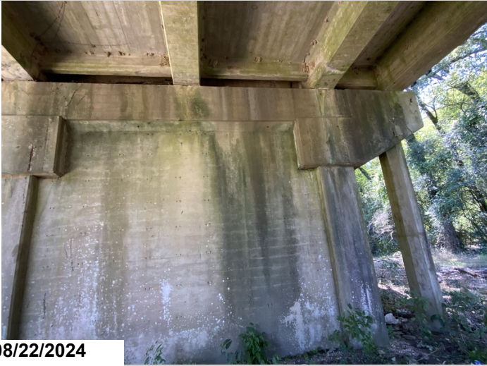
Bent 28 cap ahead right side exposed rebar 1' CS2
