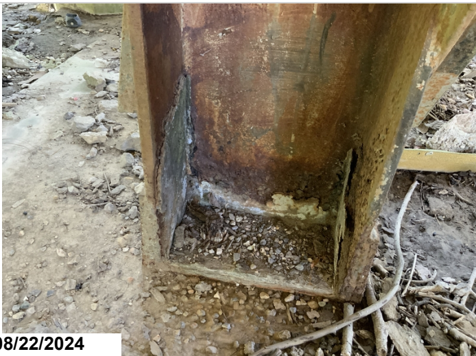
Bent 27 pile 9 1' corrosion CS3
