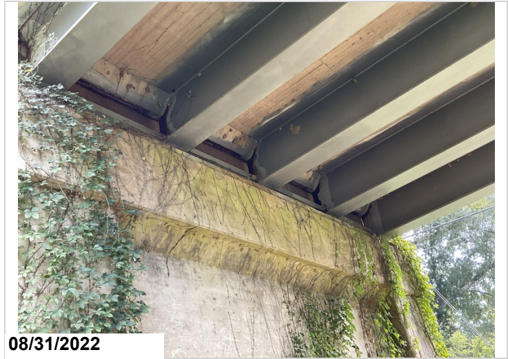
Span 30 at Bt. 31, all beam ends have active corrosion.
