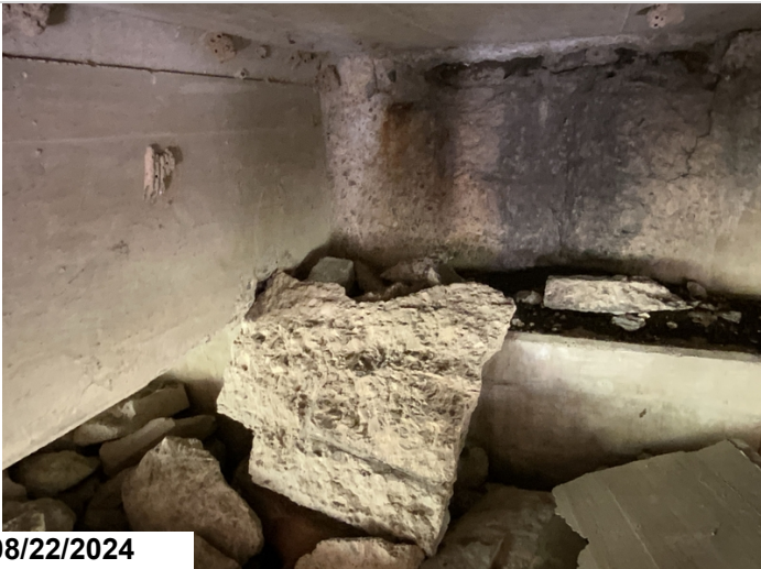
Span 1 @ abut 1 girder 1 has 1' exposed rebar CS3
