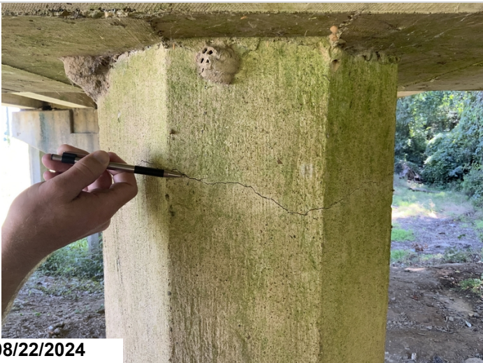
Bent 4 pile 3 cracked CS2
