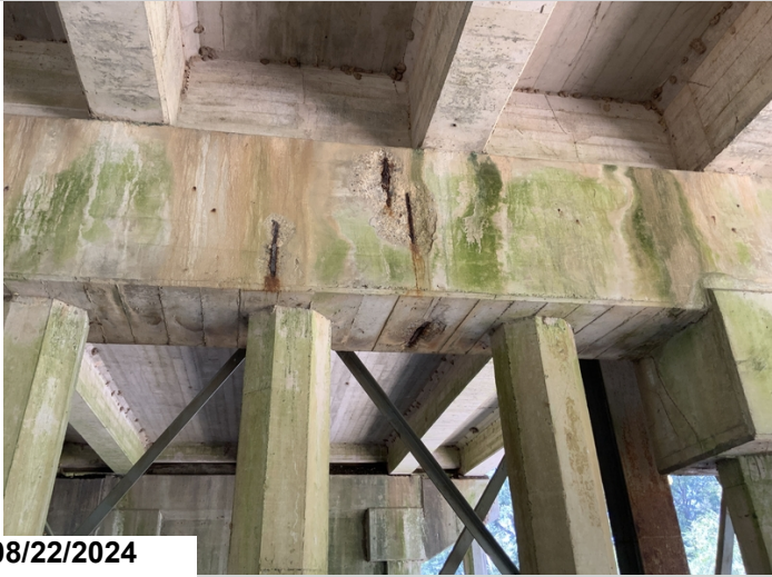
Bent 27 cap back above pile 3 has 3' exposed rebar CS3.
