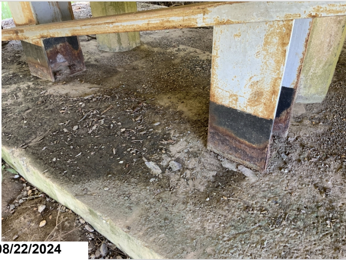
Bent 17, all 6 steel helper piles have flaking rust. 6' CS2.
