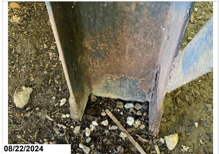
Bent 18 pile 10 flaking rust, all piles in this bent has flaking rust 1' CS2
