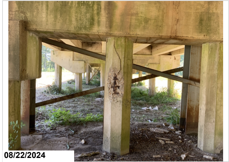
Bent 15 pile 4 exposed rebar 1' CS3
