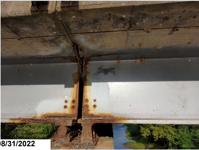
Span 29 and 30 at Bt. 30, Beam 5, beam end has active corrosion.
