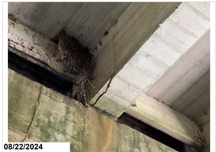
Span 23 bent 24 girder 4, delam 1'CS2
