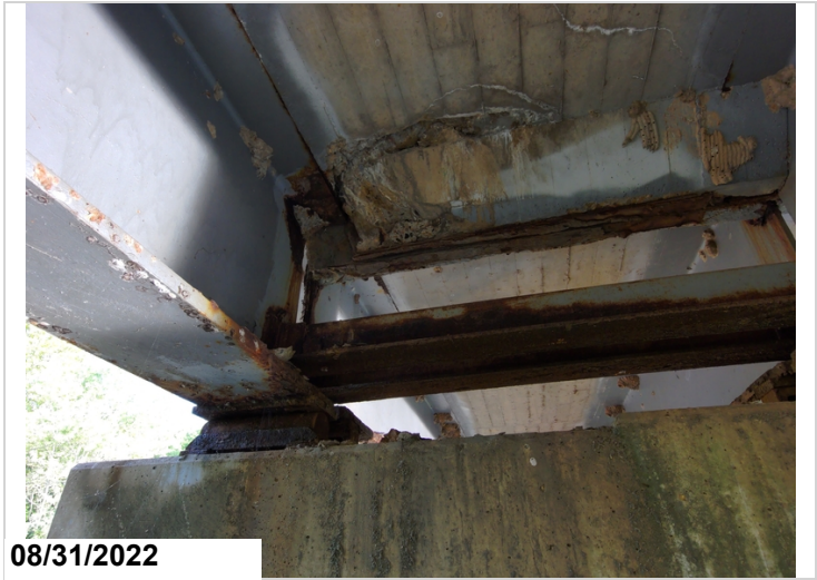
Span 29 at Bt. 30, Beam 1, beam end has active corrosion.
