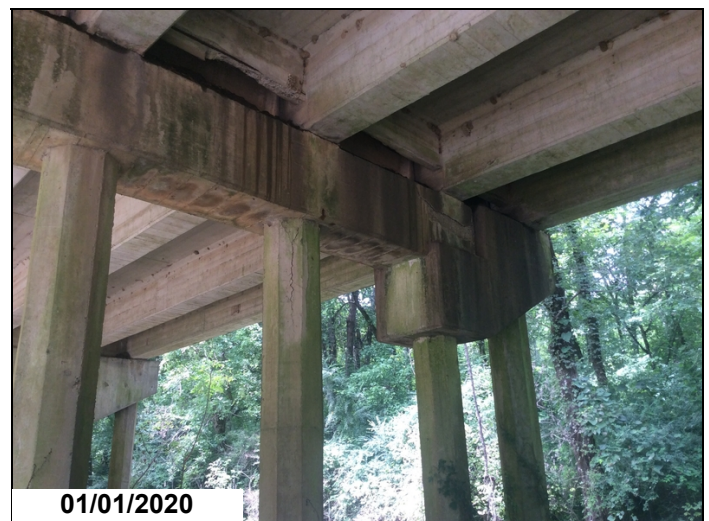
Bent 26 ahead, Pile 3 has a 3' crack that starts @ bottom of the cap & goes down.
