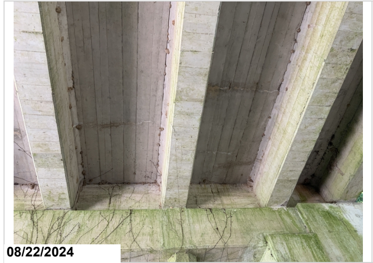
Span 23 bays 1 and 2 efflorescence 25' CS2.
