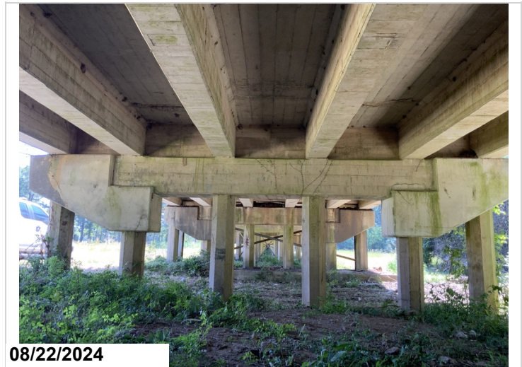
Span 16 bays 1-4 have exposed rebar, 5' CS3
