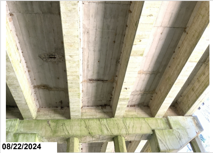
Span 22 bays 1-5 efflorescence 36sq' cs2 Bays 2 and 3 exposed rebar 4 sq' cs3
