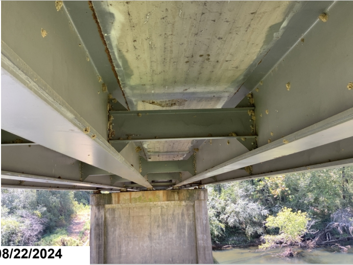
Span 30 bay 2 spall 2' CS3
