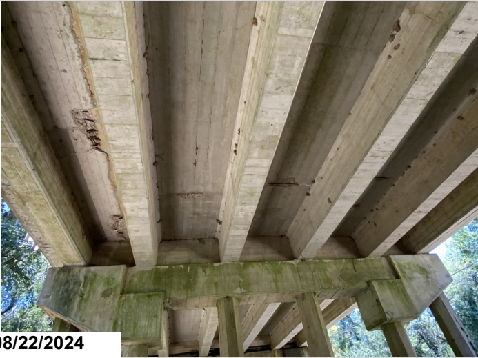
Span 24 bays 1-4 have exposed rebar, 21' CS3
