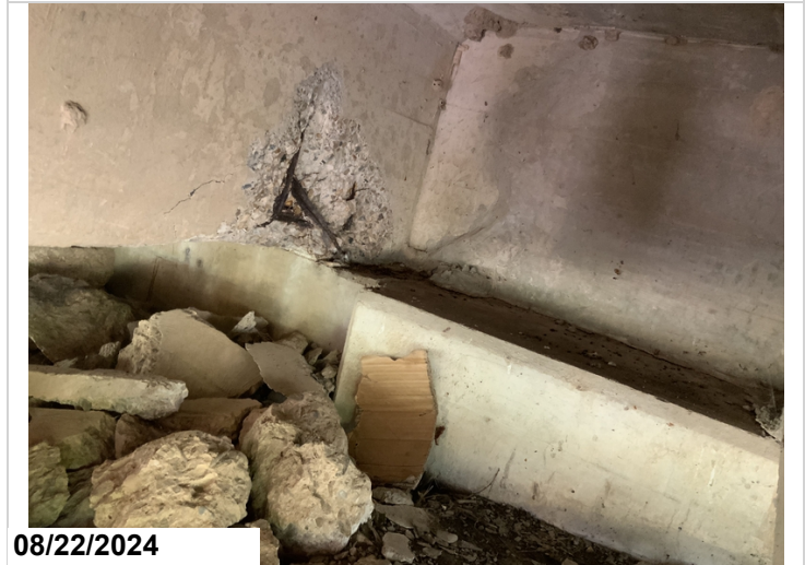
Span 1 @ abut 1 girder 2 has 1' exposed rebar CS3
