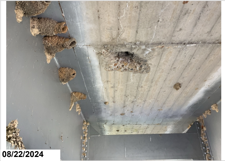
Span 29 bay 1 exposed rebar 1' CS2
