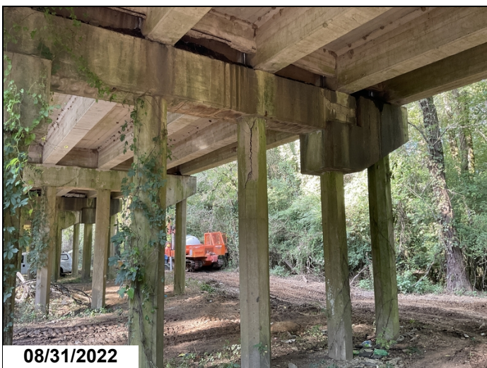
Bt. 26, pile 3 has large crack, cap has spall below girder 2.
