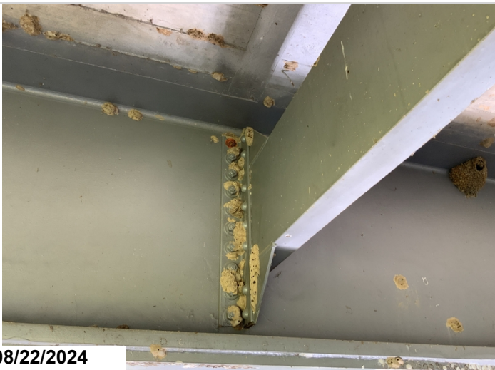
Span 30 girder 5 left at first diaphragm ahead of bent 30: missing nut.
