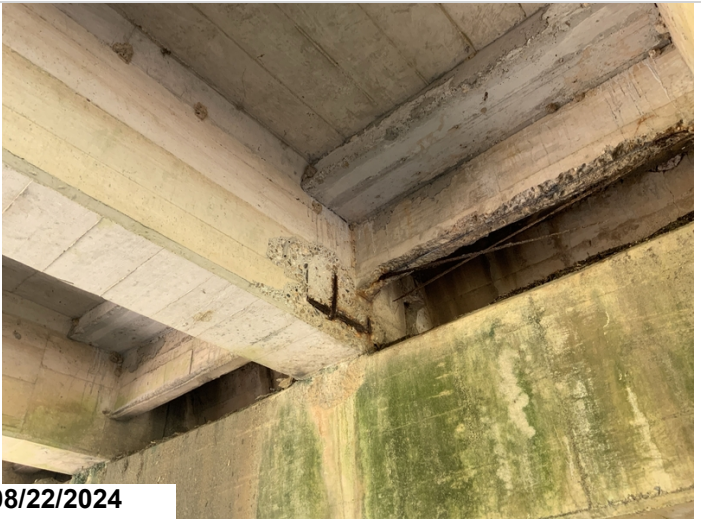
Span 12 bent 13 girder 3, exposed rebar 1' CS3
