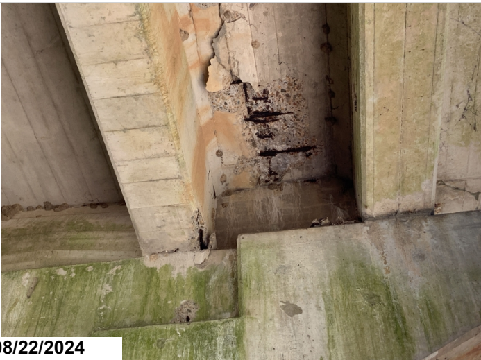
Span 25 girder 2, spall with exposed rebar cs 3
