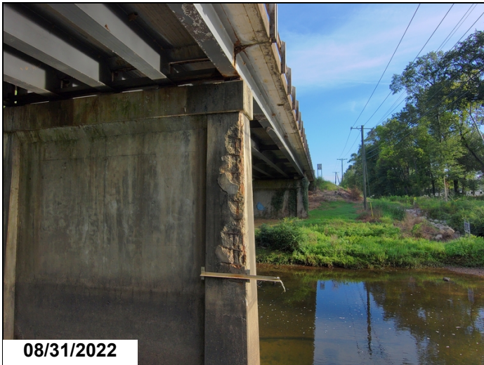
Bt. 30, column 2, spall with exposed rebar
