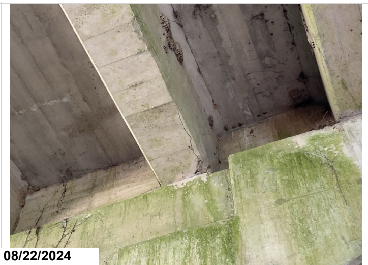
Span 23 bent 23 girder 2, delam 1' CS2
