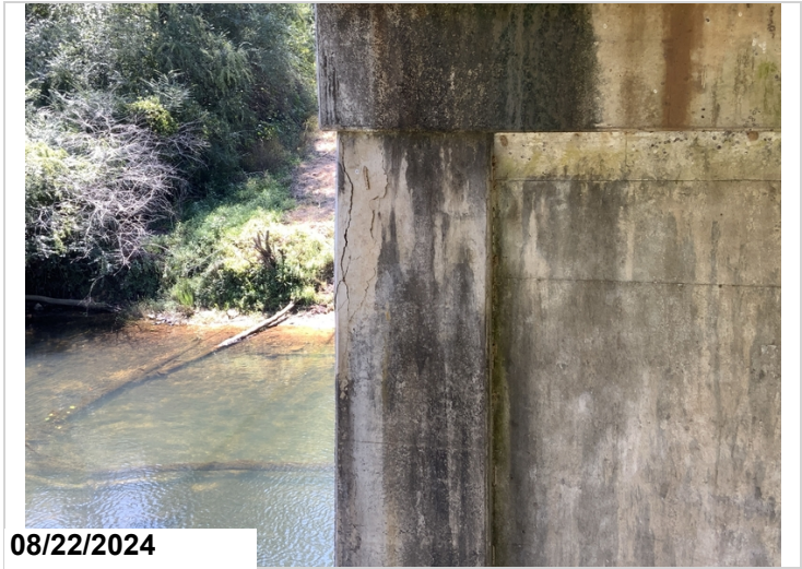
Bent 30 ahead face column 2 : large delaminating near cap CS3
